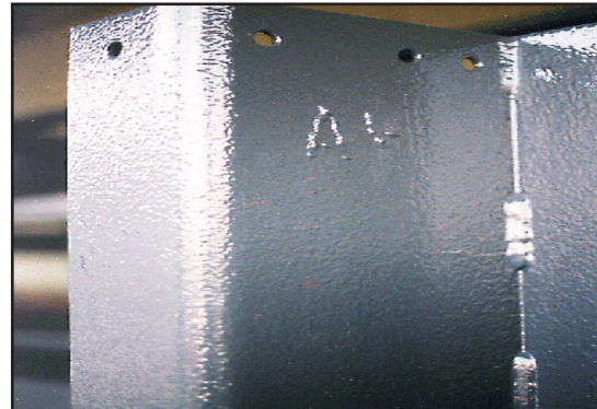
Screen supports coated with ARC 855
