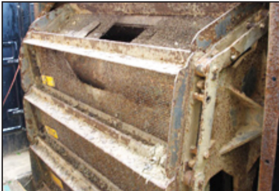
Corroded traveling screen
